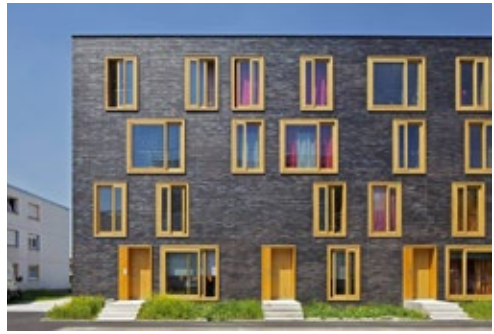
Abb. 32 23 Dwellings (2012), Bethune, Fres architectes
