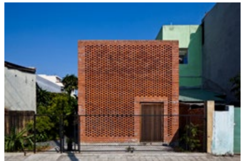
Abb. 30 Termitary House (2014), Da Nang, Tropical Studio
