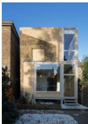
Abb. 44 House of Trace (2015), London, Tsurata Architects
