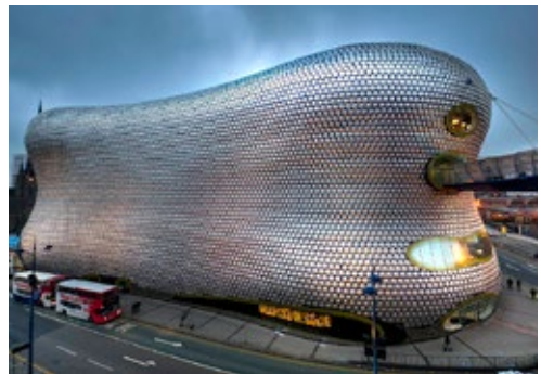
Abb. 3 Shopping Centre Selfridges Building Birmingham (2003), Future Systems
